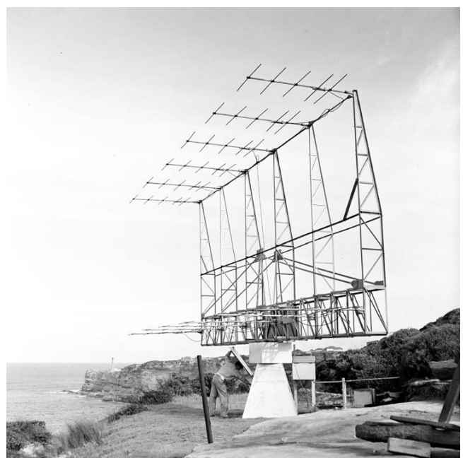
Figure 1.1: Ruby Payne-Scott, Don Yablsey and John Bolton were the first to use these Yagi antennas at Dover Heights, Sydney, Australia, in 1947. This setup was used for solar and compact radio source observations at 100 MHz.
